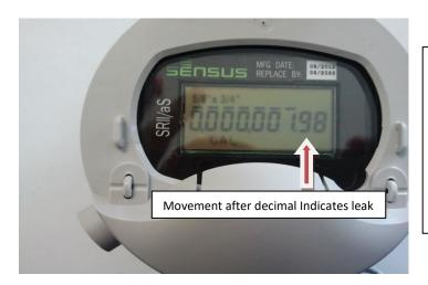
Sensus Meter- If you have a possible leak then the numbers after the decimal will be moving. Please allow 5 seconds for movement. If numbers do not appear, you may have to open & close the gray case to wake the meter up.
